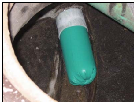
Figure 10-4 CIPP Liner Being Blown Out the End of a Lateral
