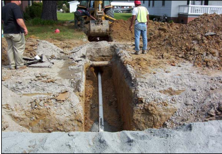
Figure 10-1 Open Trench Lateral Repair
