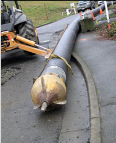
Figure 10-2 Bursting Head Attached to New HDPE Pipe
