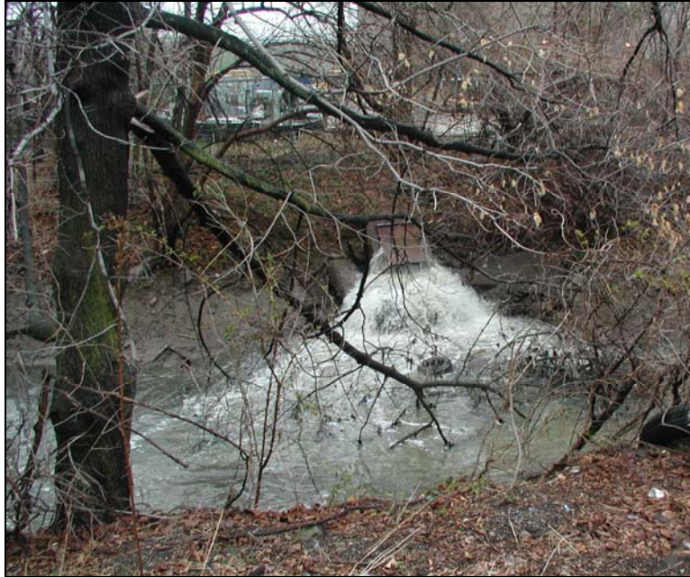
Figure 2-1 High-Flow Bypass in Delaware County
